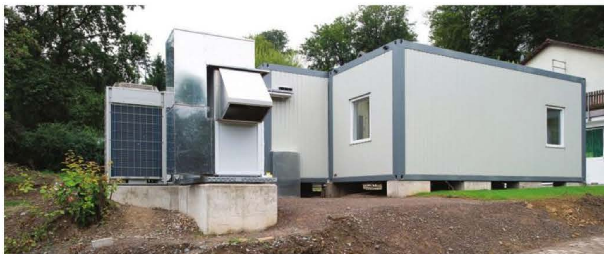
WISAG built this modular cleanroom facility for production of animal therapies at its facility in Dresden and then transported it by lorry to the client in Osterode
